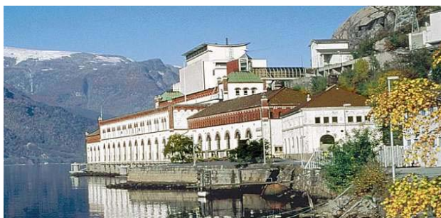
The Hydroelectric power plant in Tyssedal
